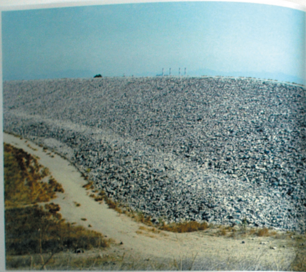
Above: View of the compacted earth fill Hansen Dam. Height from trail to top of dam is about 97 feet.
