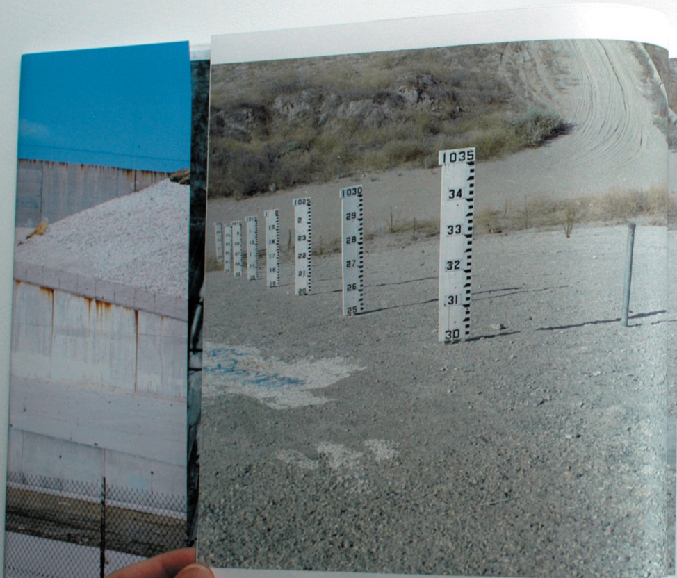
Above: Water level markers on Hansen Dam, backside of spillway. Increments are in feet above sea level.
